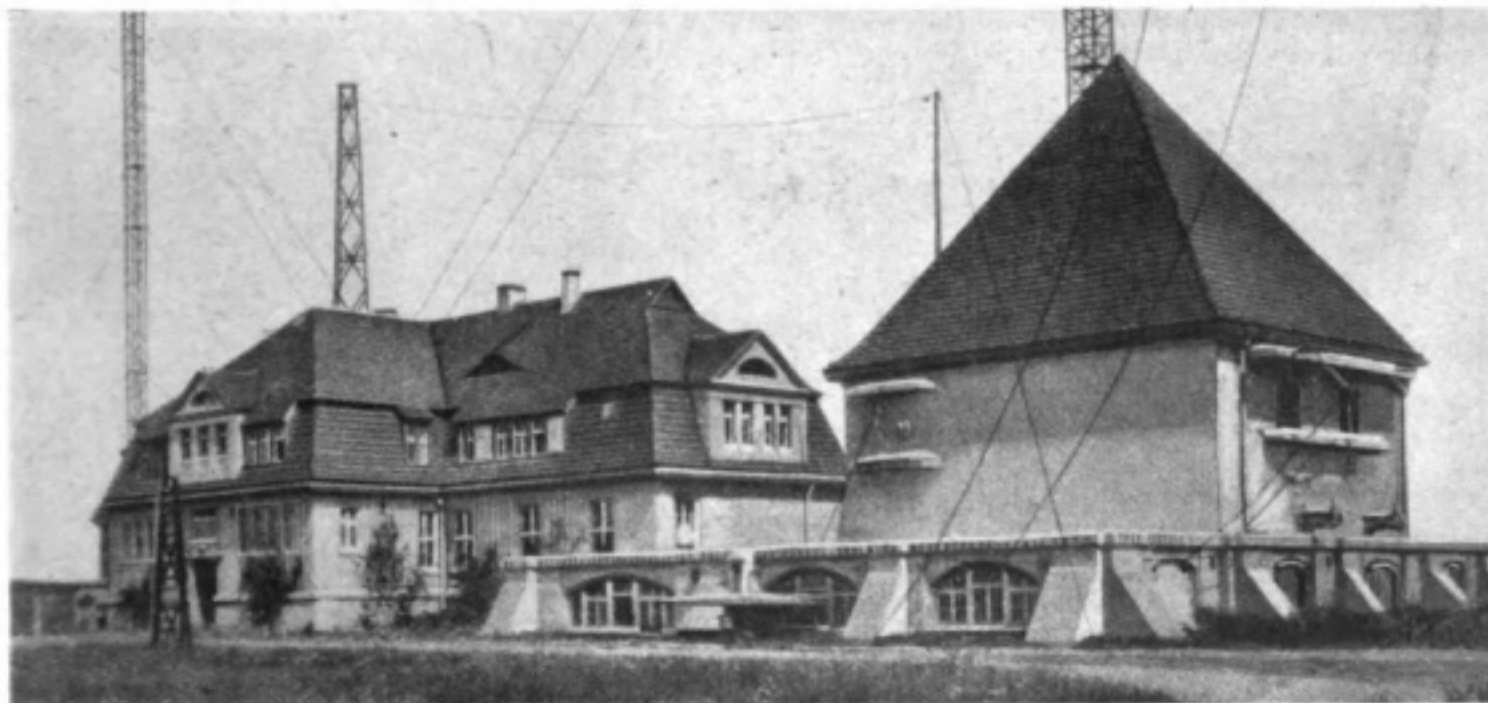
Fig. 1. The Station Buildings.
